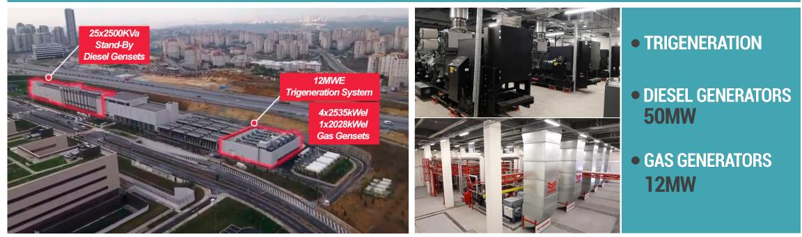
Trigeneration System with a 12MW electricity capacity, producing electricity, heating and cooling, works with diesel generators that are activated when there is an interruption in the grid, synchronously.
